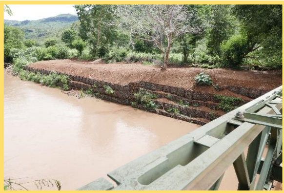
Back fill finished at bridge with gabions
